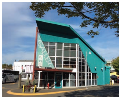
Exterior FCA gallery & offices
